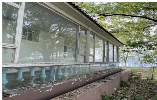
Figure 7 Current situation of the facade of the old building
