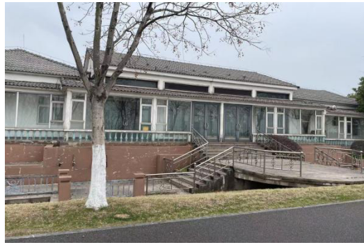
Figure 8 Current situation of the building's glass curtain wall
